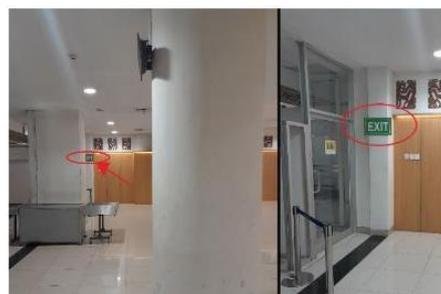
**Figure 1.** Exit sign that is covered by a pillar
