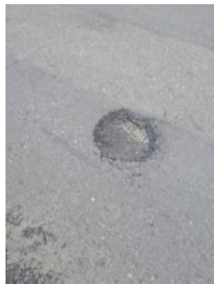
Figure 11. Hole Damage
